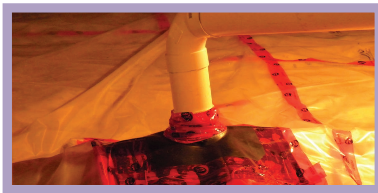
Picture 7 – Sealing the penetration through the membrane
