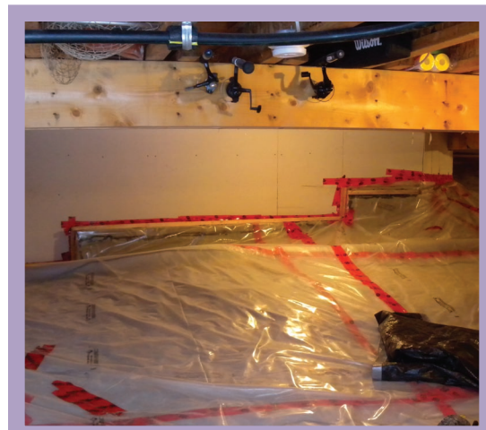
Photo 6 – Membrane and Wall Attachment
