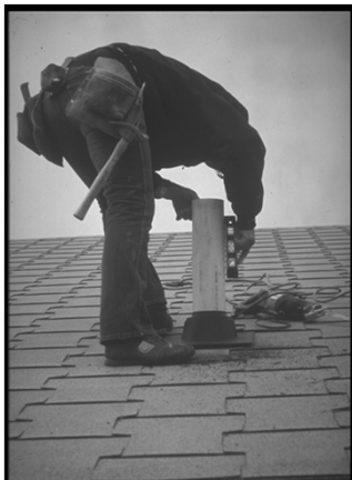
Terminate 12 inches above roof
