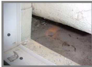
View of gap under bathtub viewed through return air duct chase
