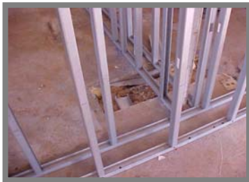
Block out for tub shown during construction
